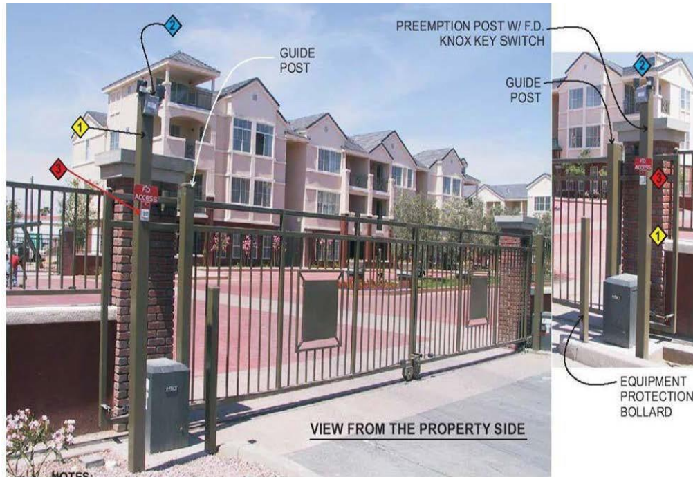
Figure 1 - Property Side of Gate
